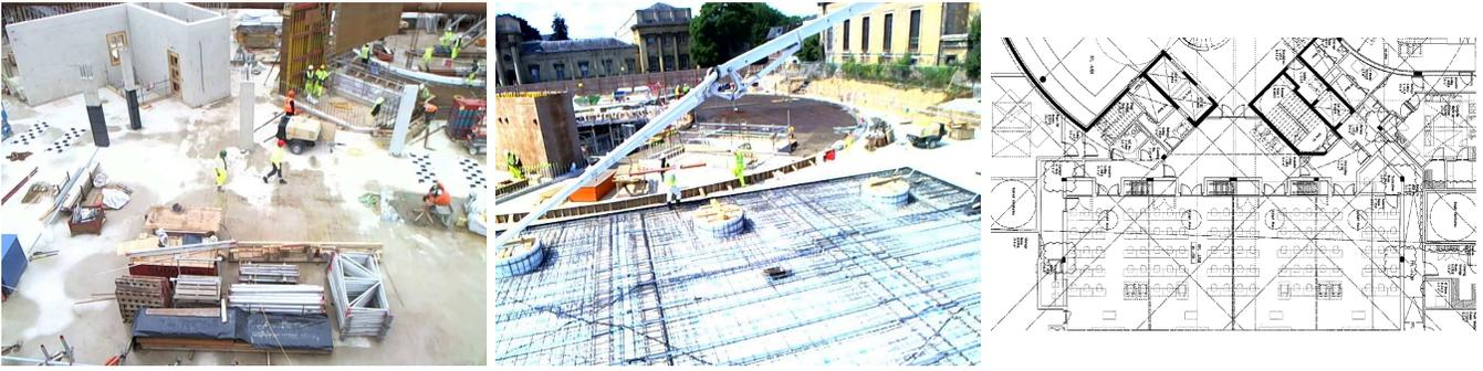
Figure 2: We have conducted tracking experiments in a construction site setting: (a) the construction site on day 1, (b) the construction site on day 36, (c) floor plan of the site. The site changes rapidly from day to day, precluding the use of positioning systems which rely on stable, long-term maps.
